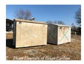
work Larry! In addition to the Cherokee signal house, we also acquired a signal house that sat in Farlington, KS. As you can tell in the photo above, all the original signal equipment remains in each signal house. Keep in mind, these buildings are made entirely of concrete and come in weighing 12.5
