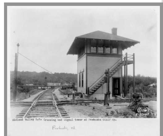
ATSF & Midland Valley crossing Pawhuska Oklahoma July 30 1927 - Construction photo. Springer Archives - Temple Texas Railroad & Heritage Museum.
